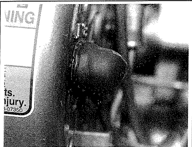
Fig. 35 . . . but should be completely sealed against the terminal base. This prevents the entry of moisture
